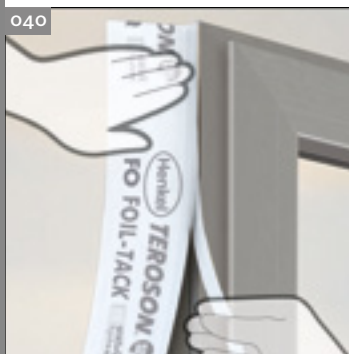
Fix TEROSON FO 50 FOIL-TACK to the frame.
