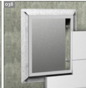
038 Install the insulation system.
