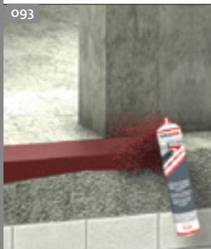
093 Pretreat mineral substrates with a primer.
