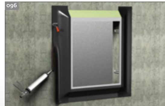
096 Seal the insulation wedge above the element.
