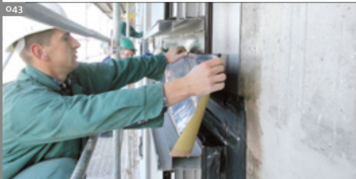
043 Remove the narrow strip of release paper and align the strip.
