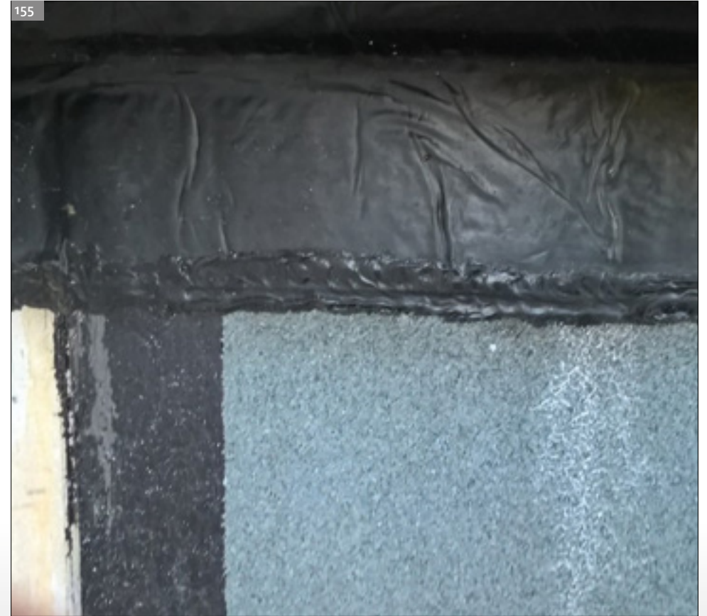
Bonding of edge seals with TEROSON AD KDS
