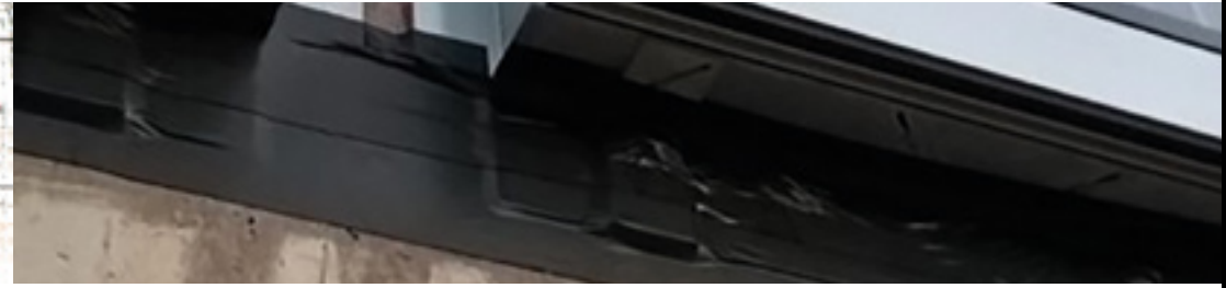
Bonding of edge seals
