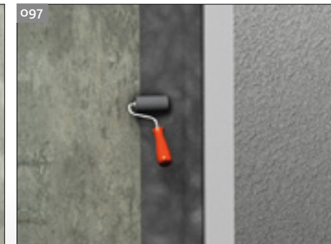
097 Press the sealing strip down with a rubber roller.
