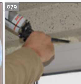
o79 Foam-filling of horizontal joints
