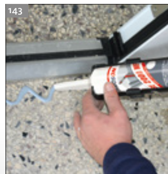
Apply the adhesive bead.
