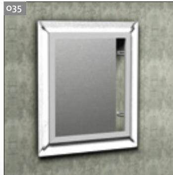
035 Fix the window frame in the insulation layer.
