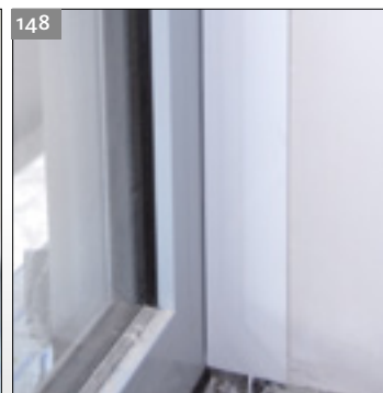
Joint-covering profile after installation
