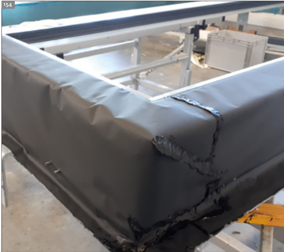
Bonding of sealed seams with TEROSON AD KDS
