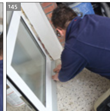
Press the rail down to the surface.
