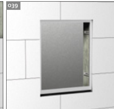
039 Facade after completed ETICS installation.
