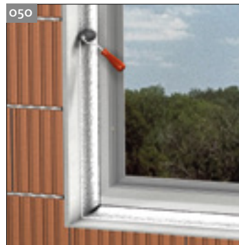
050 Press the strip down with a hard rubber roller.
