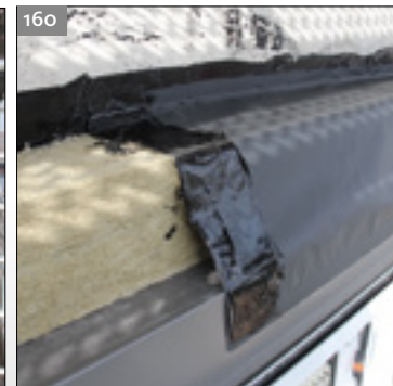
160 Seal the insulation wedge with TEROSON FO 3 membrane.
