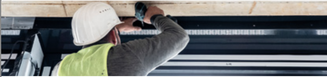
Sealing of facade panels
