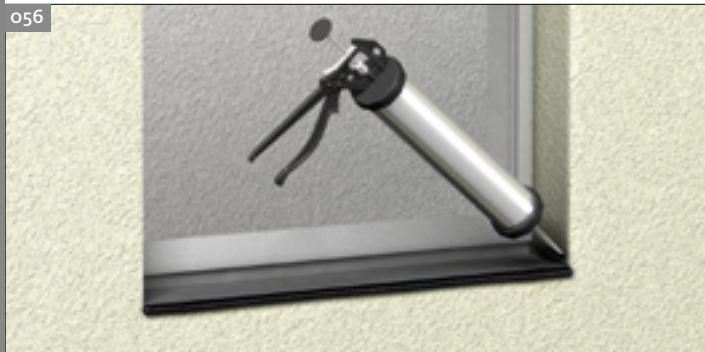
Lateral sealing of the strip with adhesive paste
