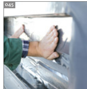
045 Manually press the strip down without blisters before using a hard rubber roller.
