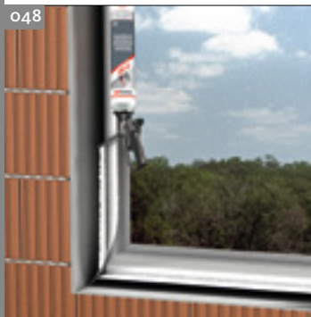
048 Fill the window connection joint with a foam sealant.
