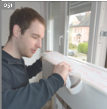
051 Position the sealing strip along the roller shutter box
