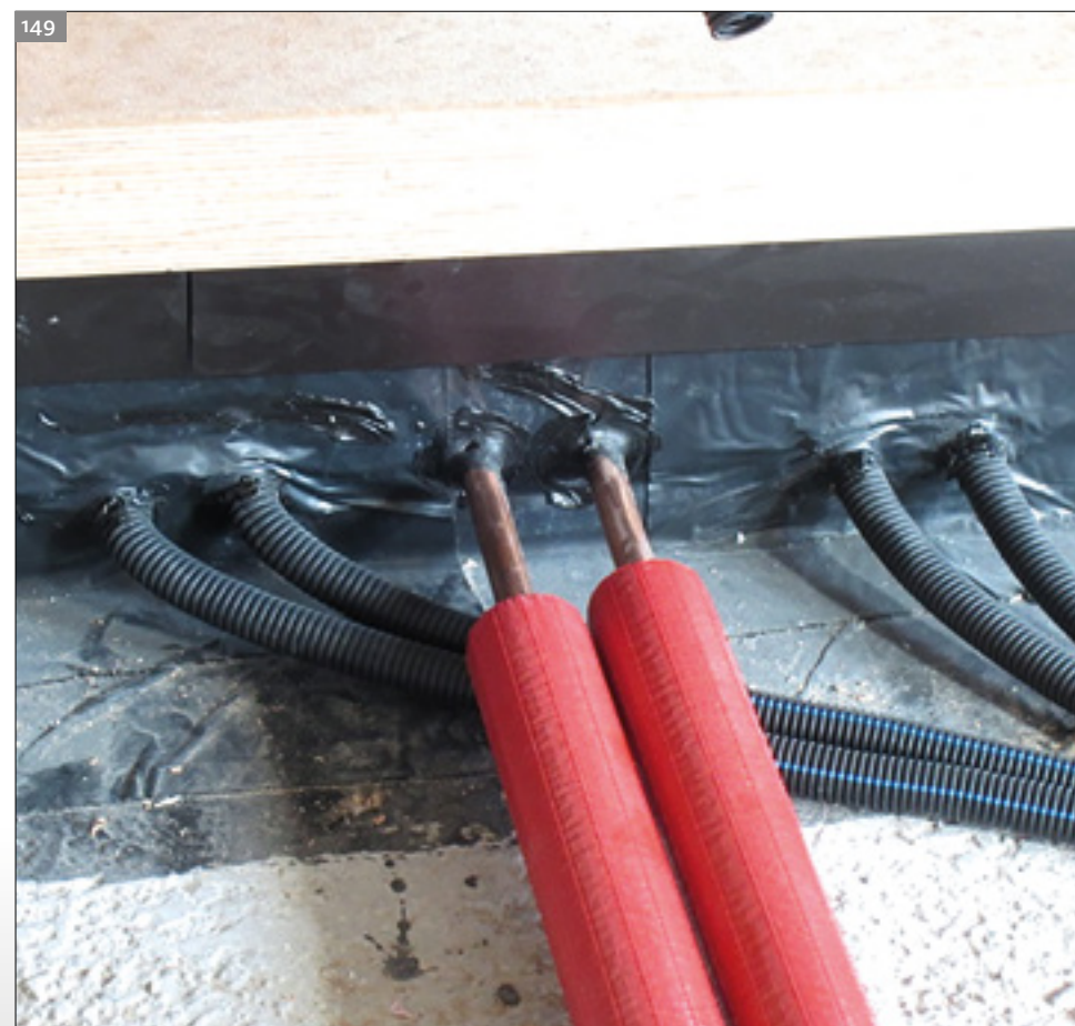
Bonding and sealing of penetrations with TEROSON SE 2000 MF and TEROSON FO 150 FOIL-TACK M+S
