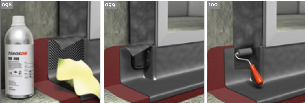
098 Pretreat the bonding area with TEROSON SB 450 primer.
